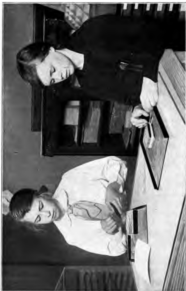
FIG. 20. Correct method of tying up type
